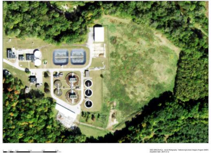
Waste Water Treatment Center
