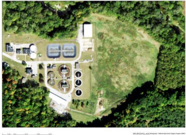
Waste Water Treatment Center
