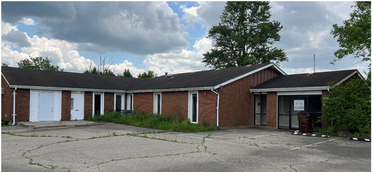
Existing Building Rear (Parking Lot Entrance)
