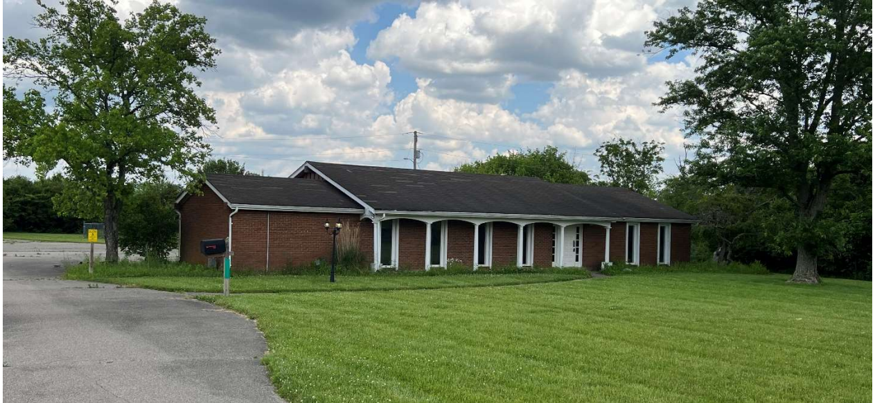
Existing Building Facing College Corner Pike
