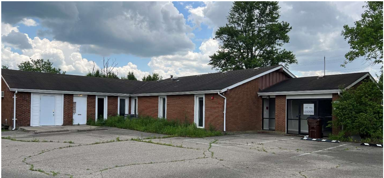
Existing Building Rear (Parking Lot Entrance)
