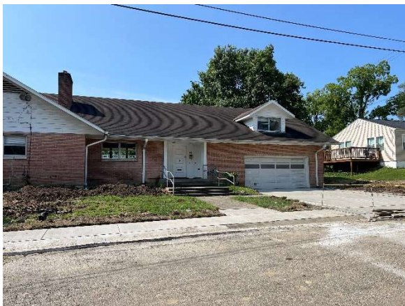
Existing Garage & Driveway
