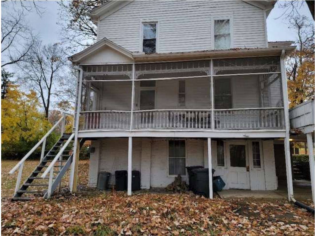
Historic photo of rear porch (Unsure of when stairs were relocated)
