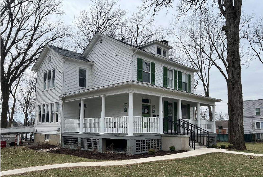
Corner of Spring & South Campus showing refinished steps & new Guardrails
