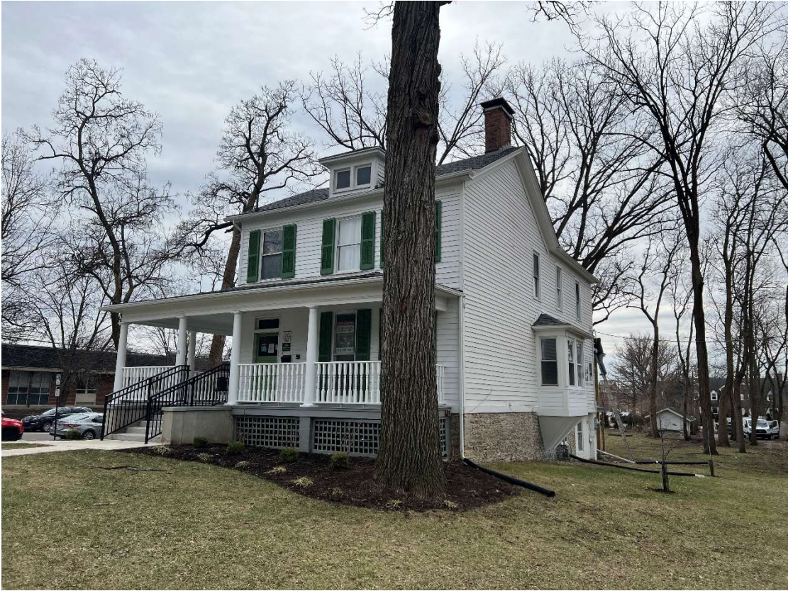
North face of the residence, showing the repaired Bay & Porch Improvements
