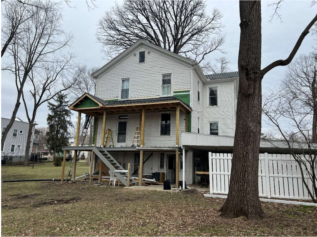
In progress photo showing reconstruction of rear Porch Roof
