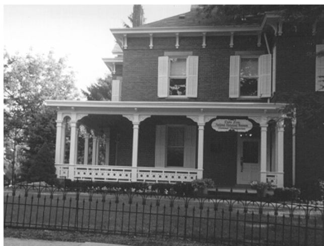
A very nice example of a well maintained porch.
