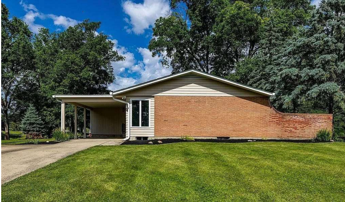
Front of House showing Existing Carport
