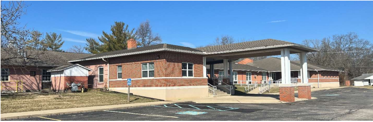
Existing Main Lobby Entrance from South
