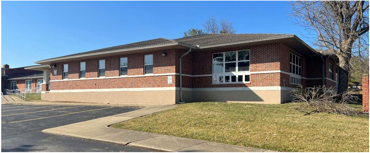
Existing Building from Entrance Drive
