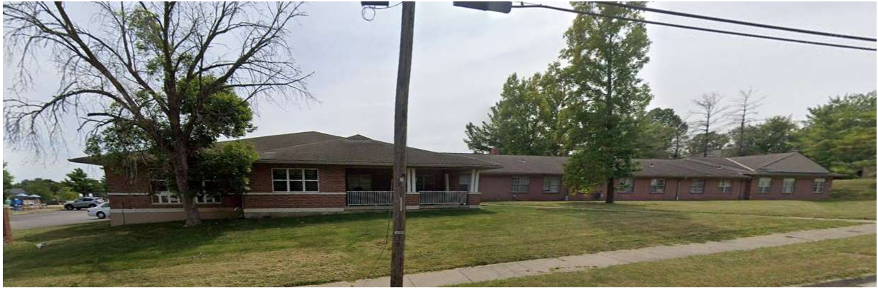
Overall Building from Fairfield Road
