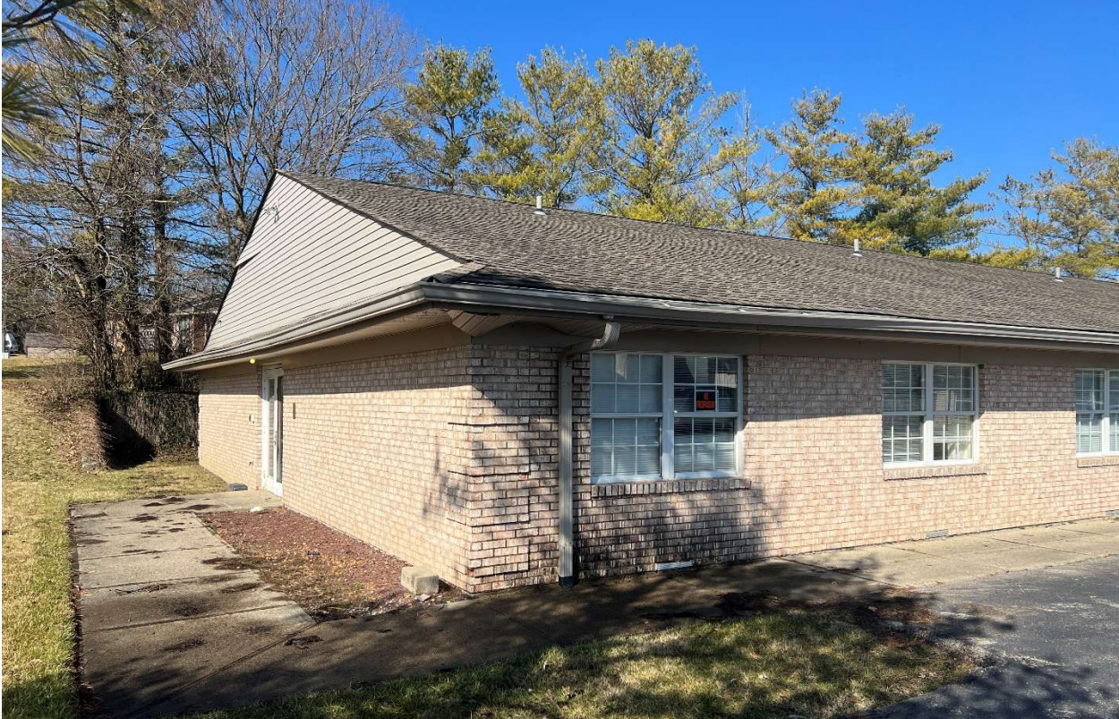
South Exterior – showing typical Brick & Windows
