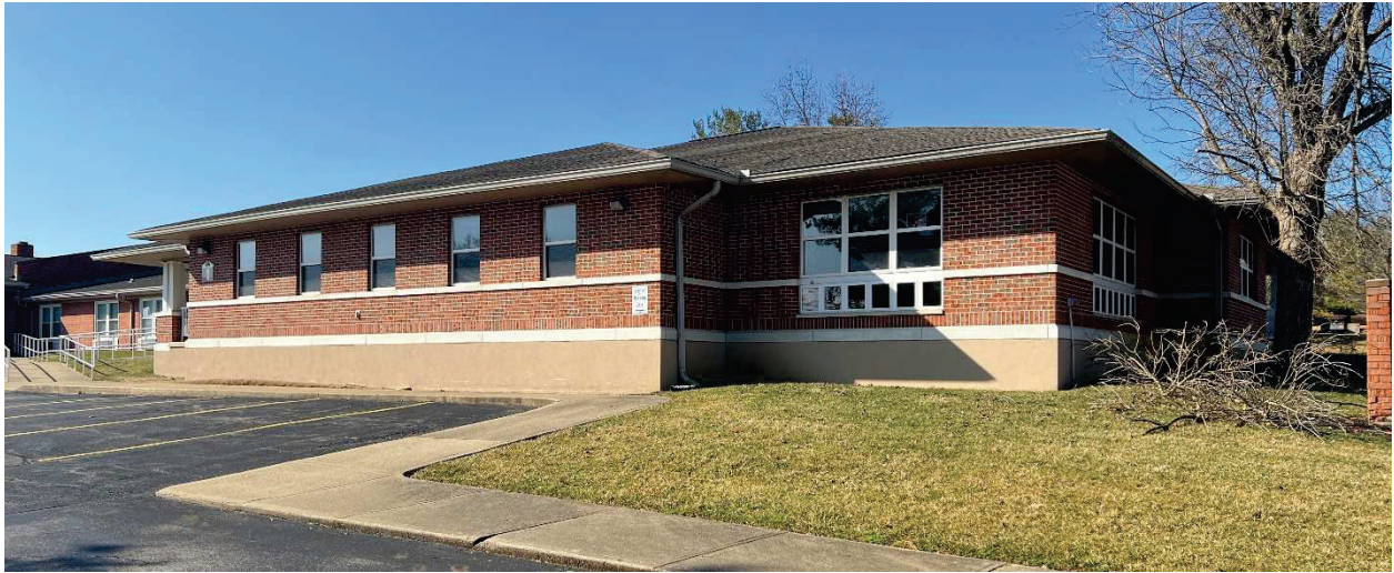
Existing Building from Entrance Drive
