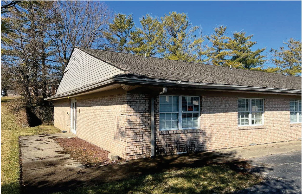
South Exterior – showing typical Brick & Windows
