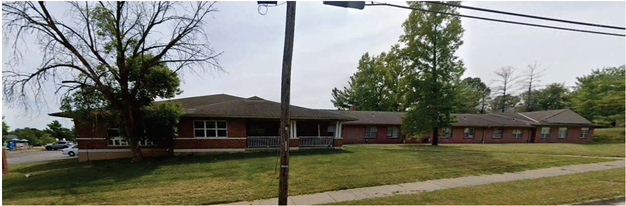
Overall Building from Fairfield Road
