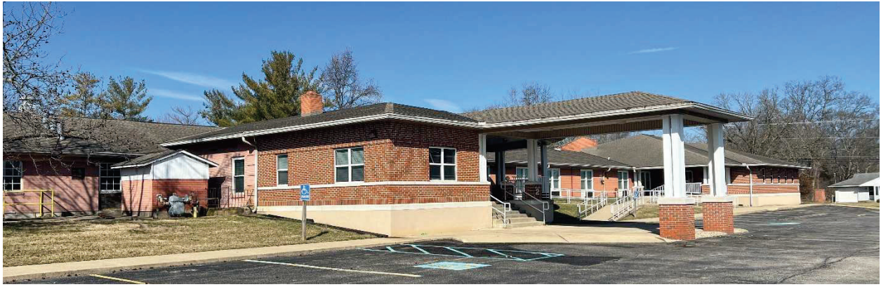
Existing Main Lobby Entrance from South
