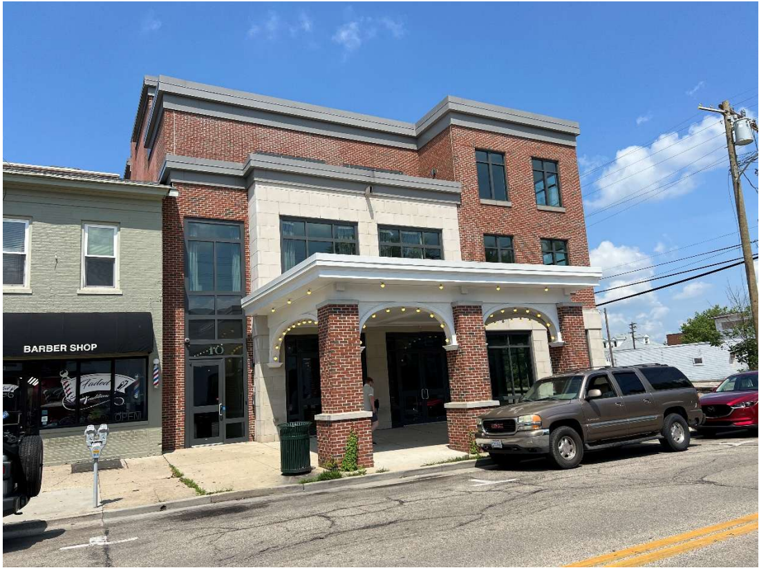
Front Façade Facing Beech Street
