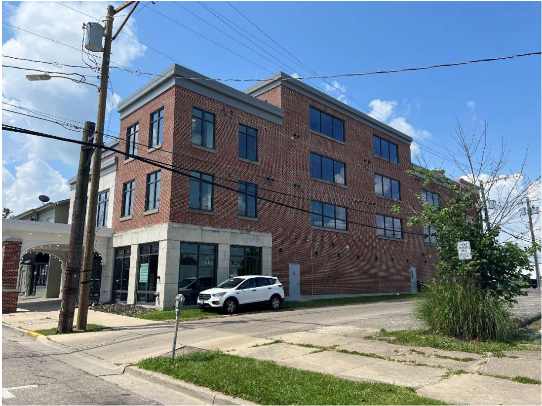
Front Façade & North Side Facing Alley
