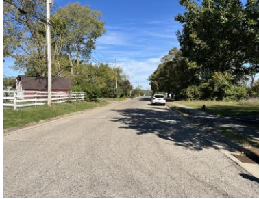
Hester Road looking north. 5234 Hester Road is on the near right.
