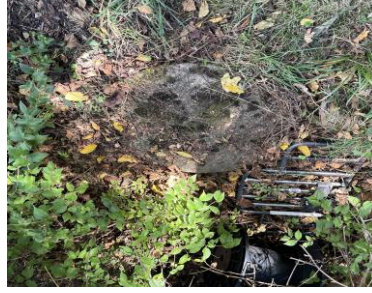
Concrete lid, grass area, 100 ft from Hester Road left of center.
