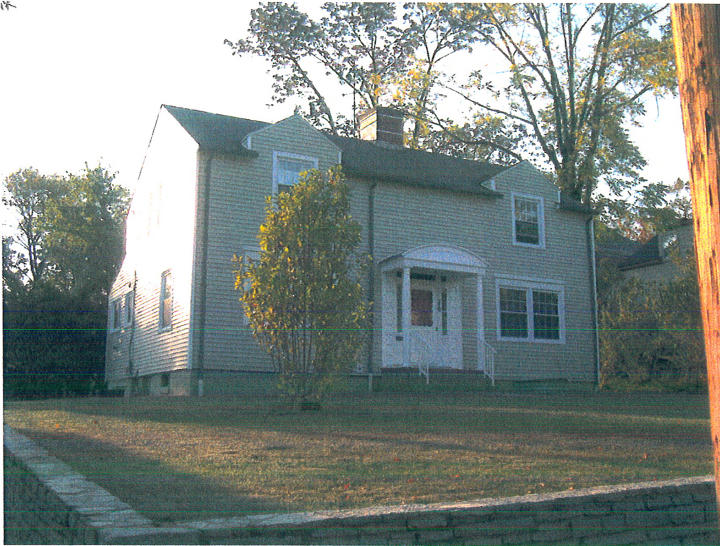
Existing Residence from Poplar Street
