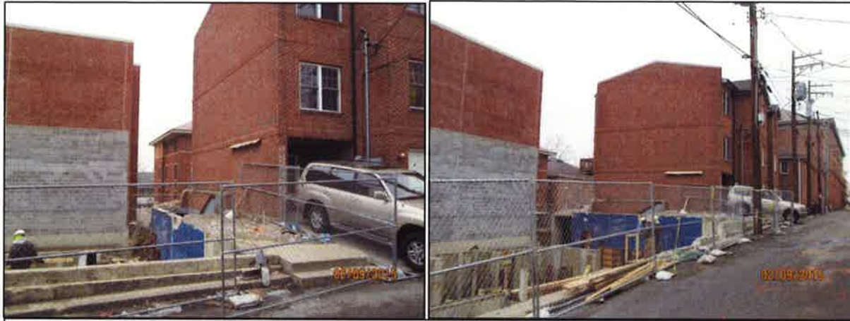
Pictured above are photographs of the current adjacent property construction project. The building at right of both photographs is the subject property proposed for reduction in lot size.
