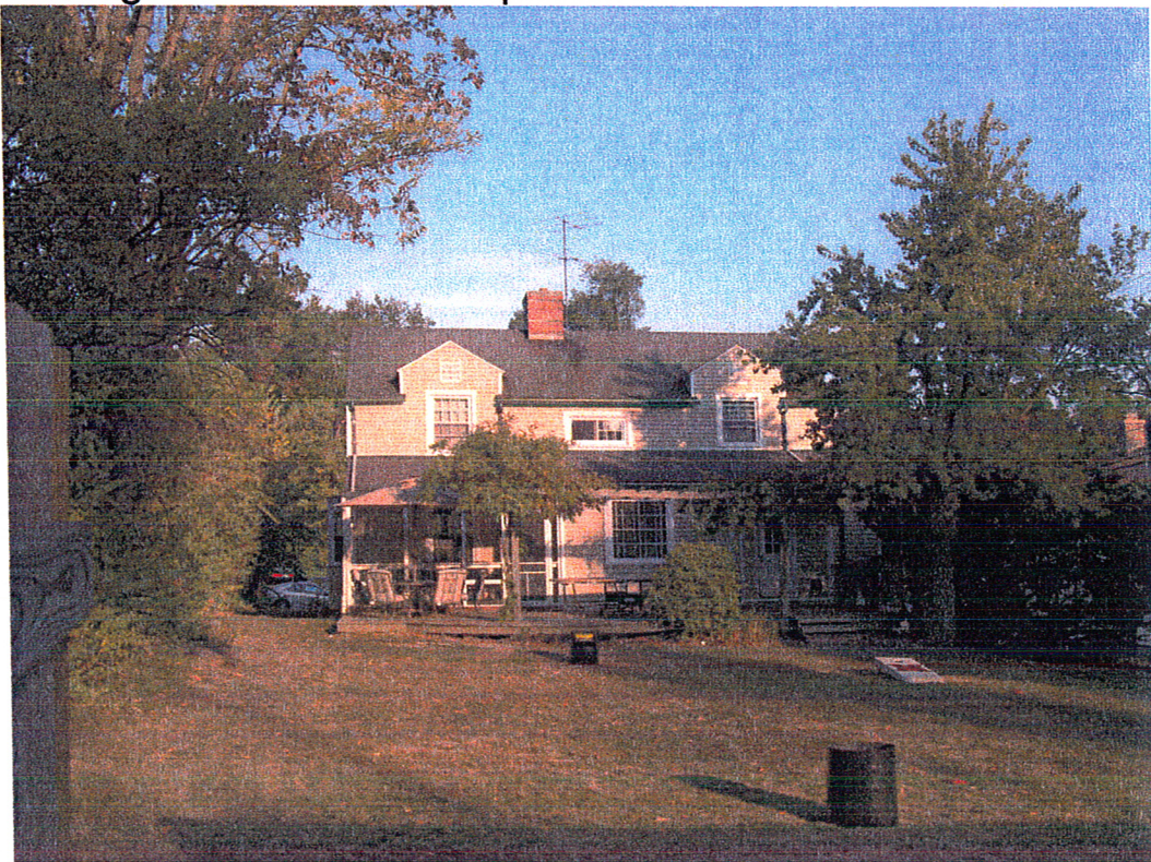
Existing Residence (Rear from Alley)
