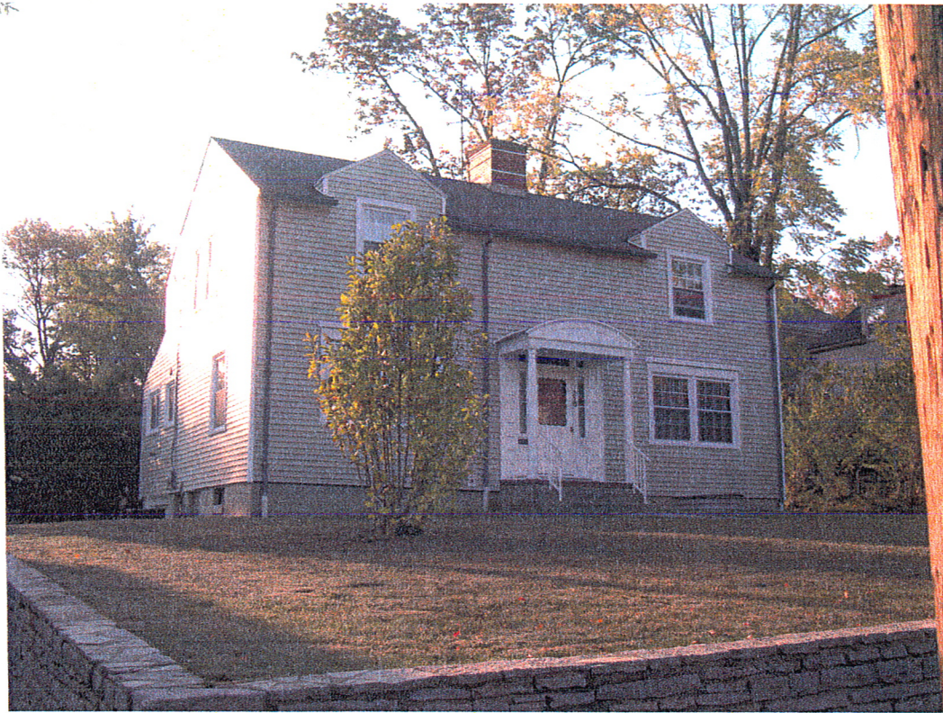
Existing Residence from Poplar Street
