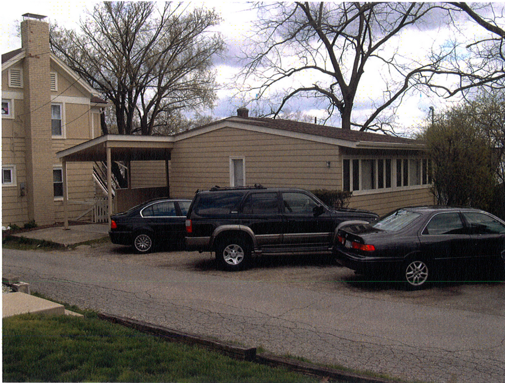
Existing "Addition" to rear
