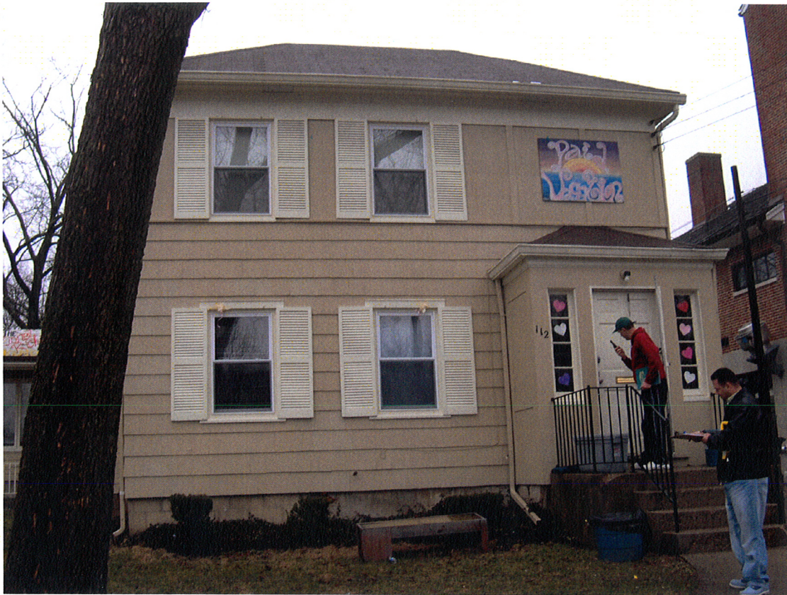
Existing Building, facing Poplar Street
