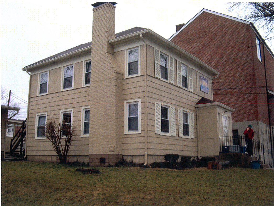
Existing Building with Church in Background
