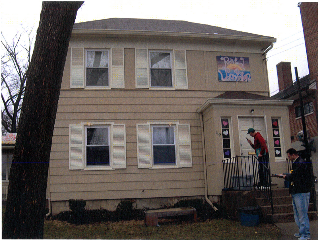
Existing Building, facing Poplar Street
