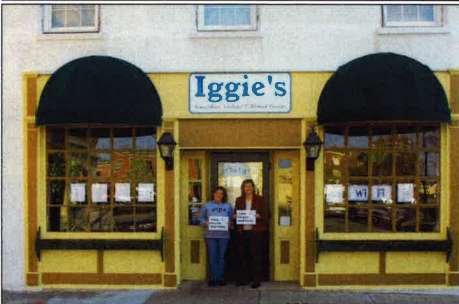
2009 photo of the façade most recently occupied by Nails Depot. Note, three historic window openings on 2 nd floor. [48 E. Park Pl.] ←
