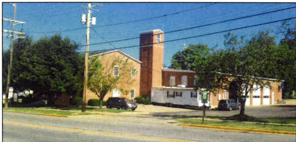
View of current fire station from Southeast
