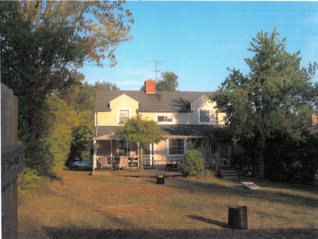
Existing Residence (Rear from Alley)
