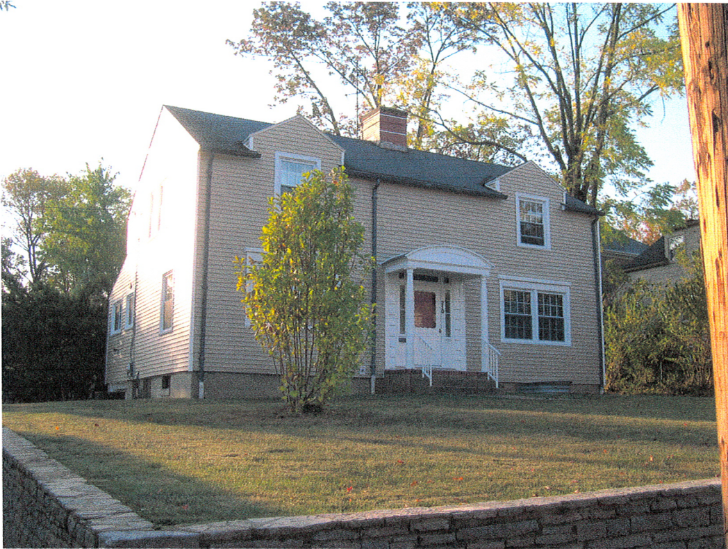
Existing Residence from Poplar Street
