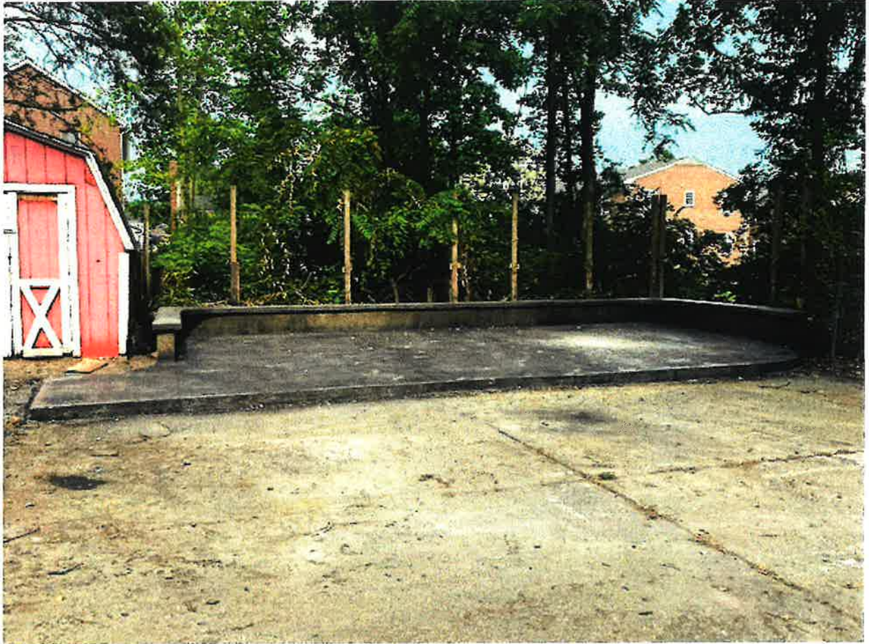
Concrete patio poured July 2021
