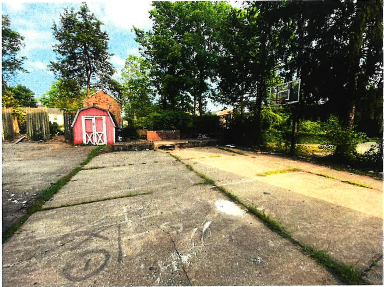
Prior wooden deck in place for several decades
