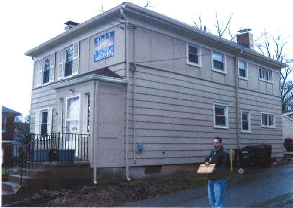
North Side Encroaching on Alley Right-of-Way
