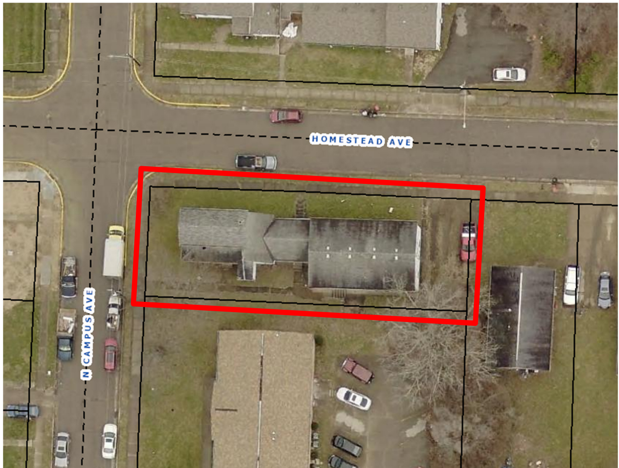
Area Map Showing Existing Structure to be removed
