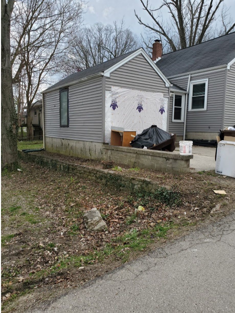
View of Former Garage & Existing Retaining Walls
