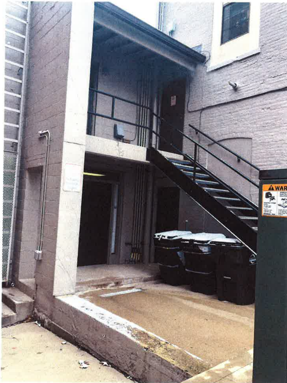
Existing Rear Entrance
