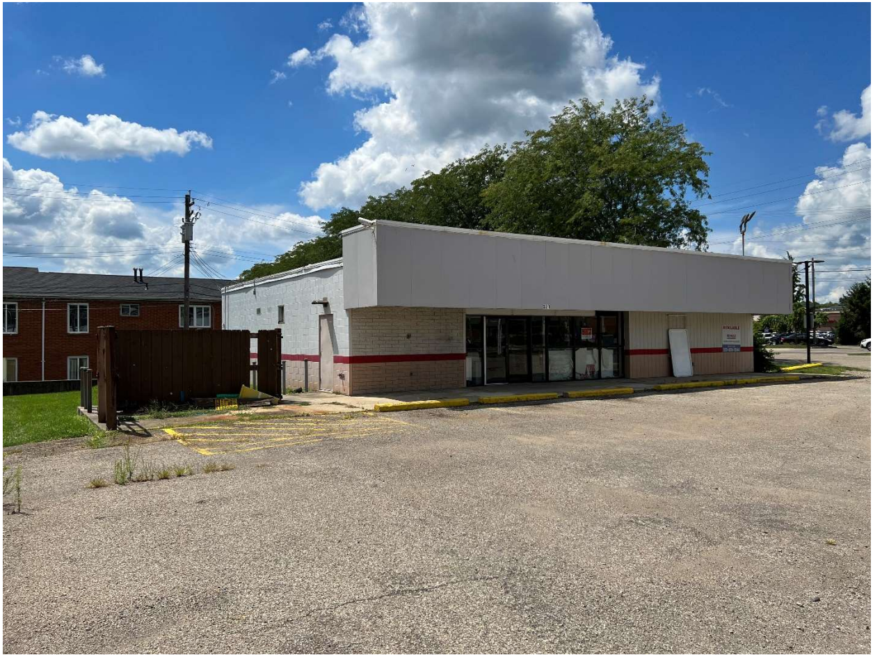
Existing Building showing existing trash area to be relocated.
