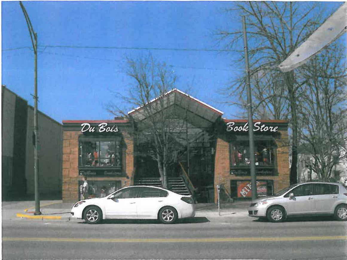
PREVIOUS BUILDING SHOWING SIGN TO BE RE-USED
