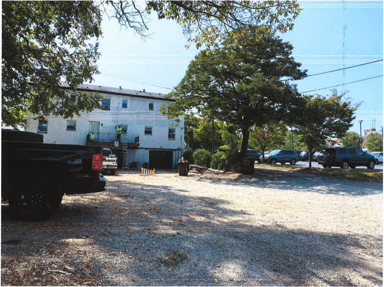
Vacant Lot from Northeast Showing lower level garages and existing Tree & retaining wall
