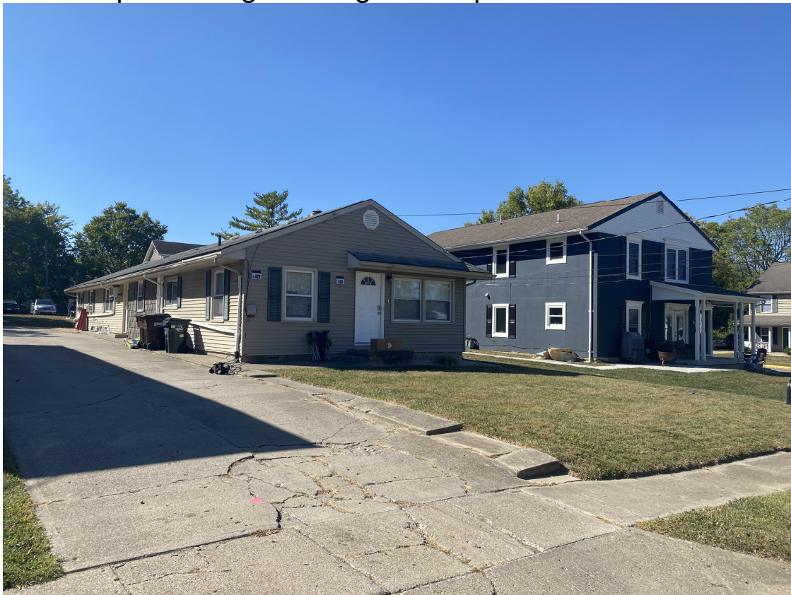
Existing Single Story Structure
