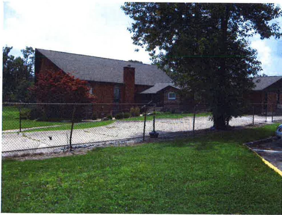
7) View from the northeast property corner facing southwest.
