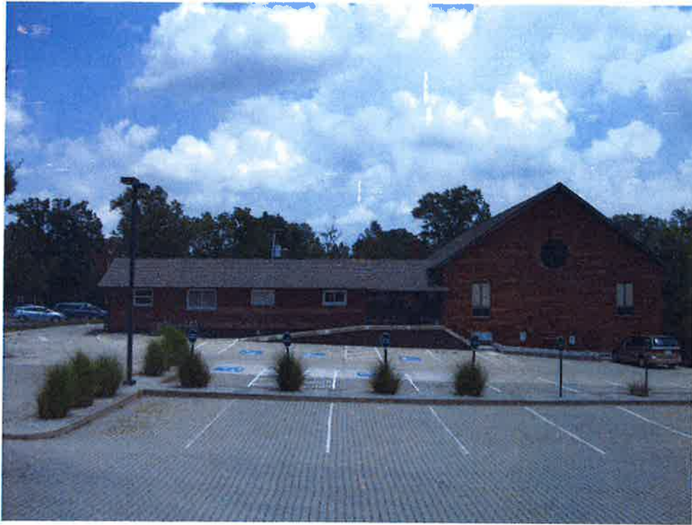
13) View from the west property line facing east.
