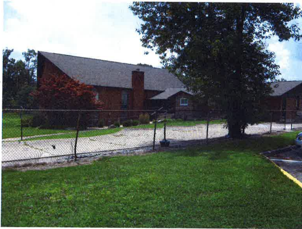
7) View from the northeast property corner facing southwest.
