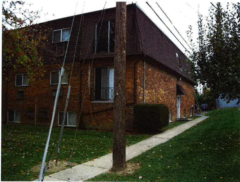
View from the northwest property corner facing southeast towards existing building #1
