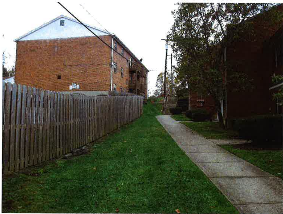
View from the southeast property corner facing southwest along the south property line and building #6
