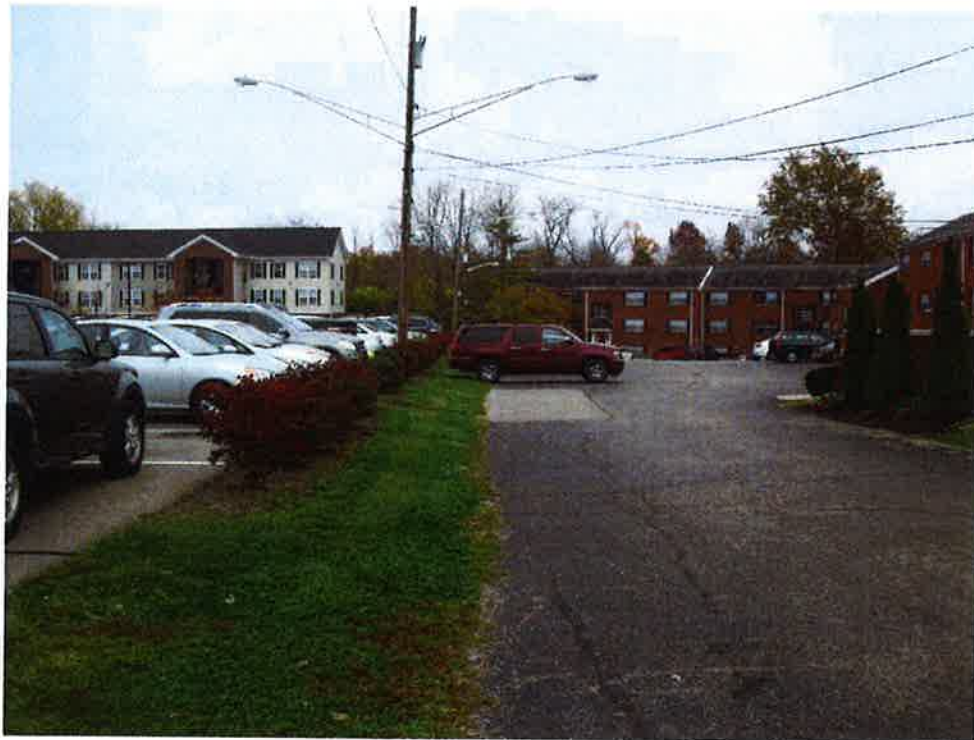
View from the the north property and entrance of building #5 facing east.
