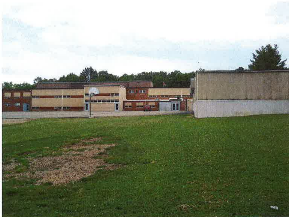
View from the north play field facing south.
