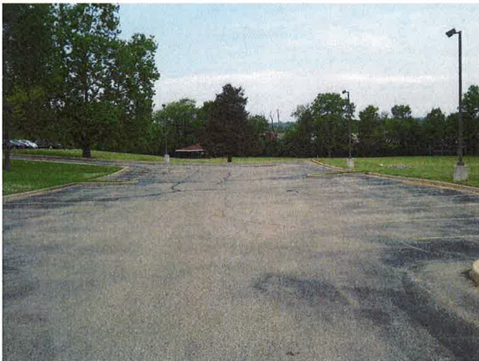
View from the center of the entrance drive of the east parking lot facing north.
