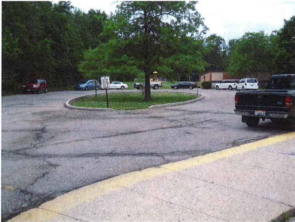
View of the entrance loop.
