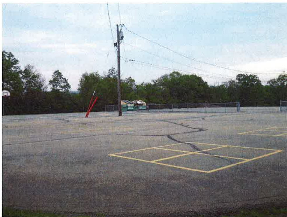
View from the north side of building facing northeast.
