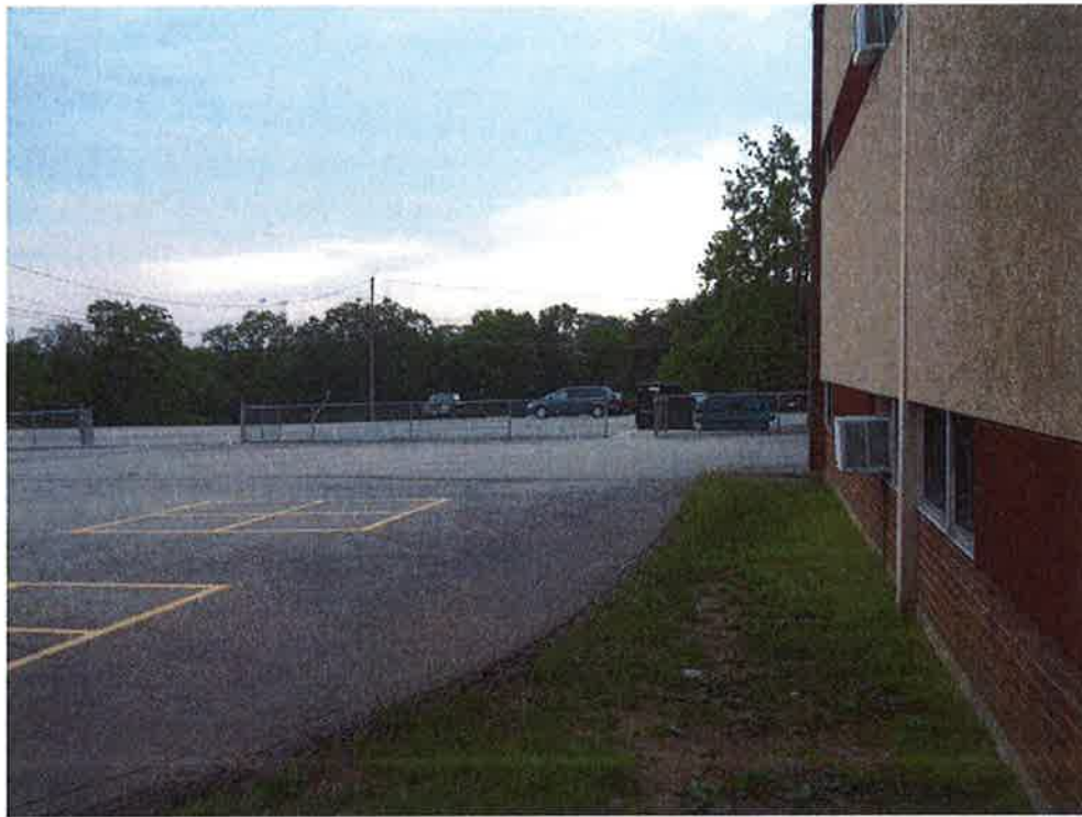
View from the north side of building facing east.
