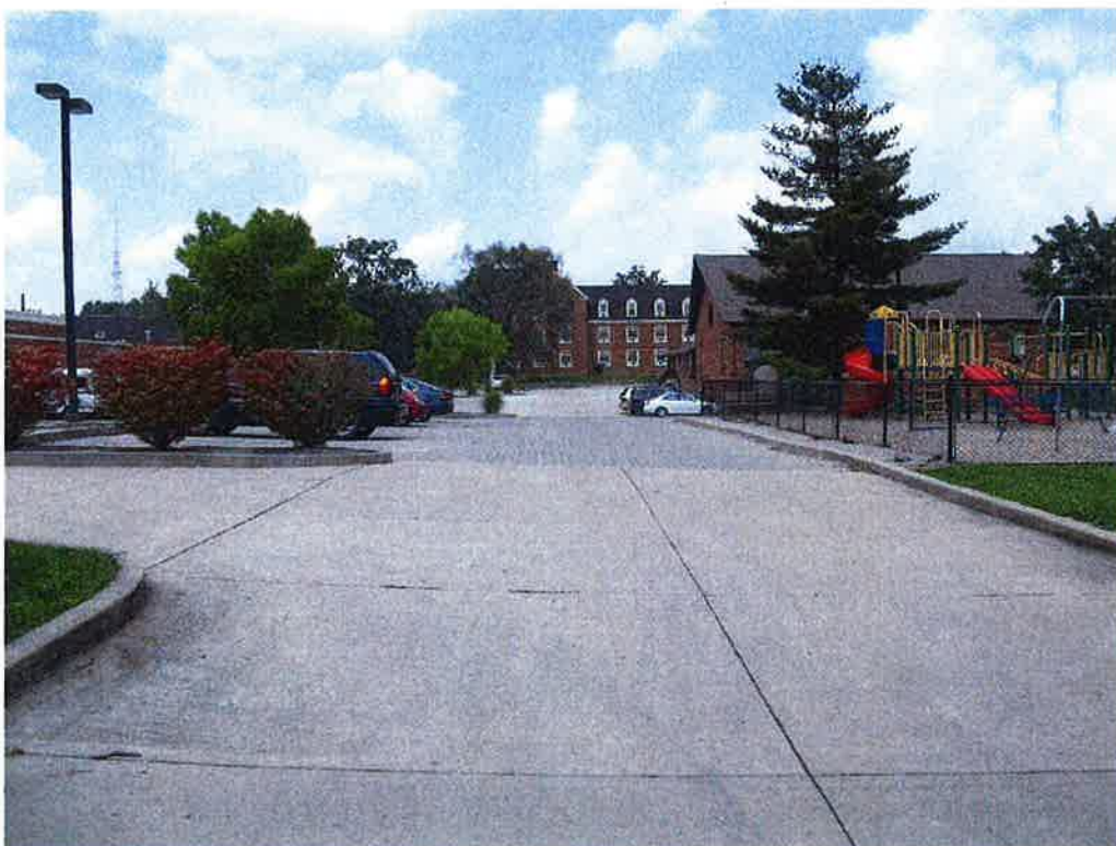
18) View from the south property line along E. Chestnut St. facing North.
