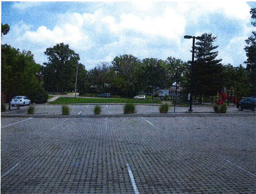
14) View from the west property line facing east.
