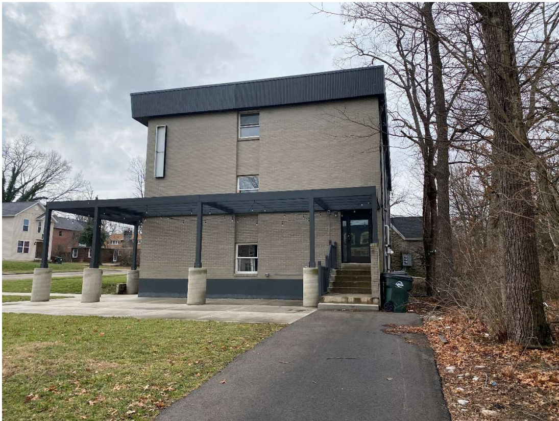
Existing Trash Area
