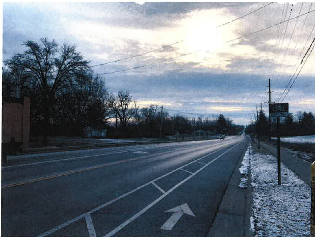
Site from North
