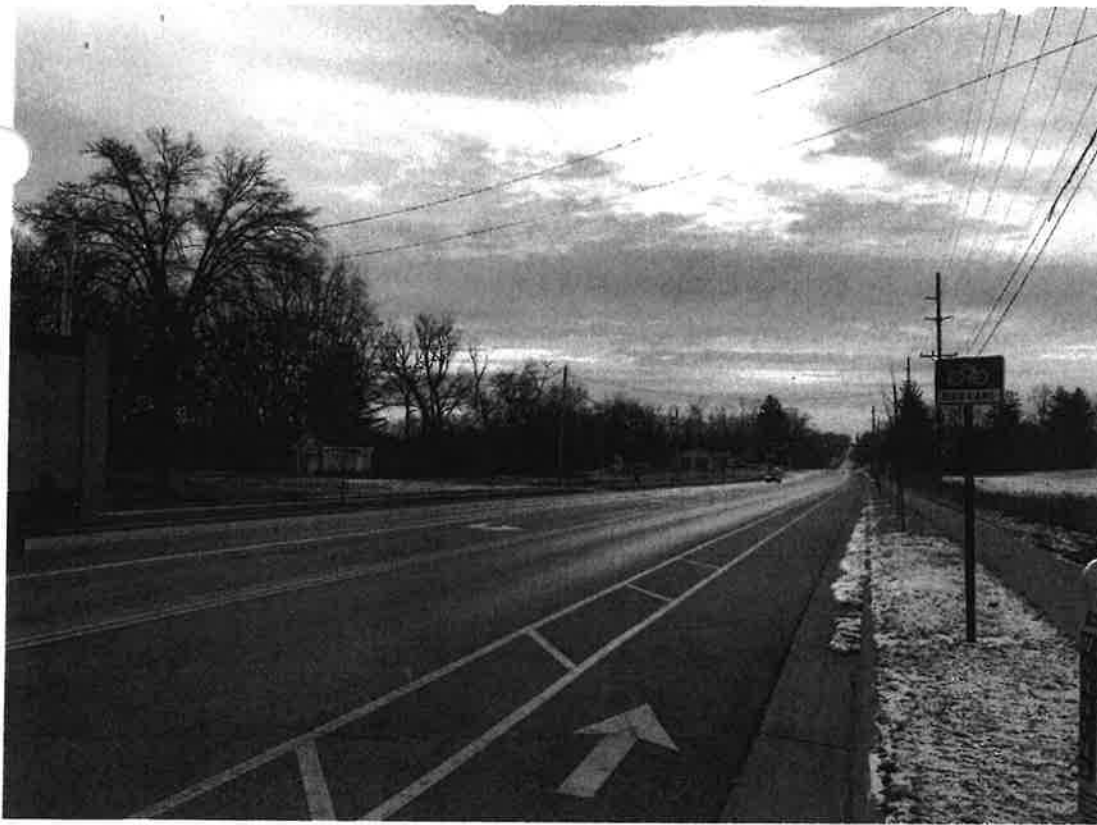
Site from North
