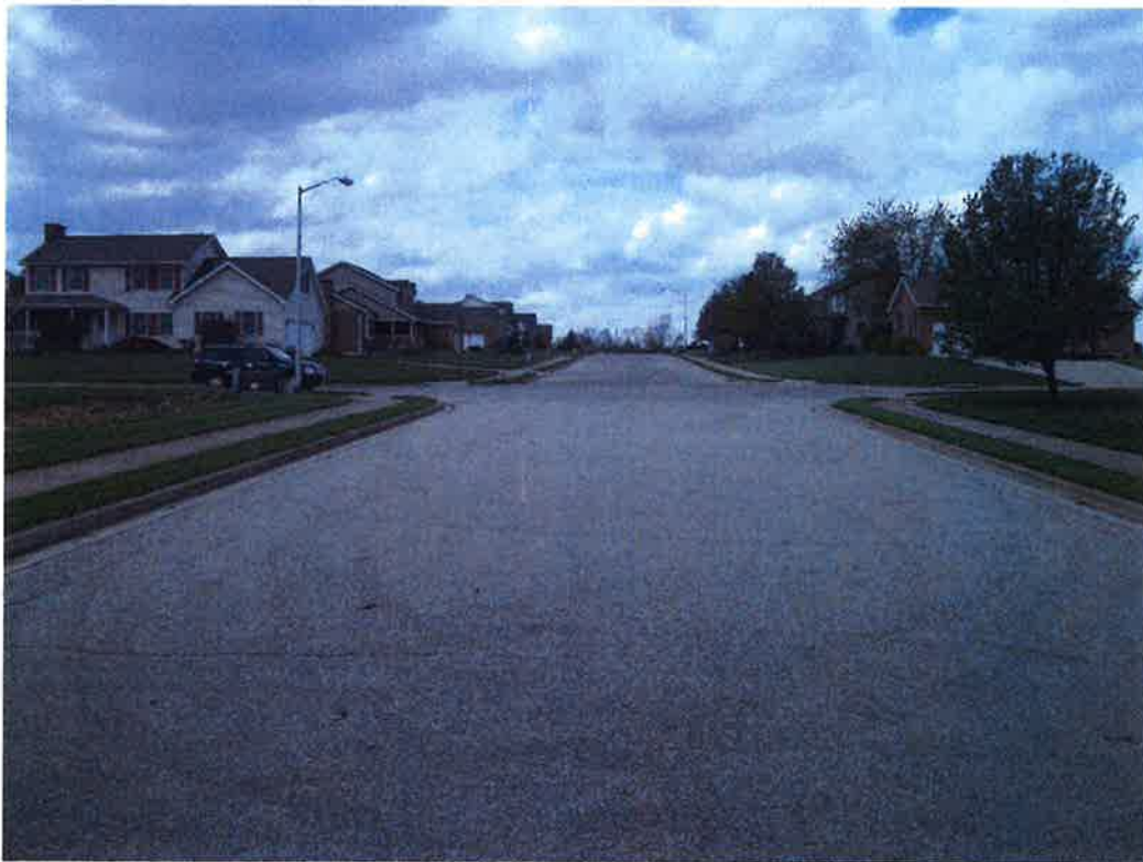
View from the center of Savannah Drive at the West property line looking West.
