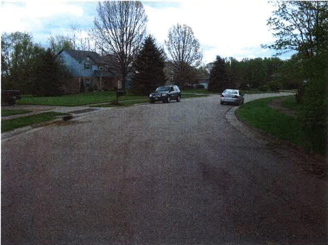
View from the center of Country Club Drive looking Southeast.
