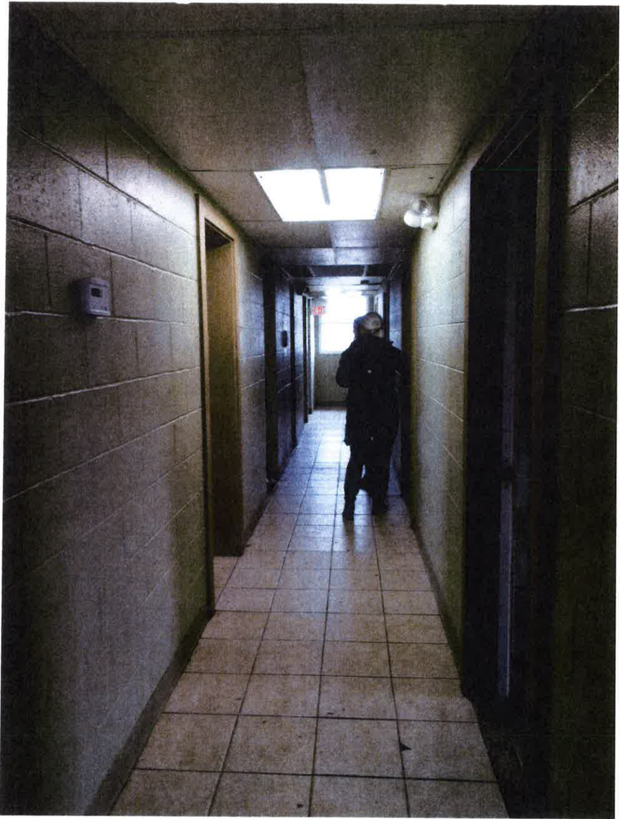
Second Floor Hallway
