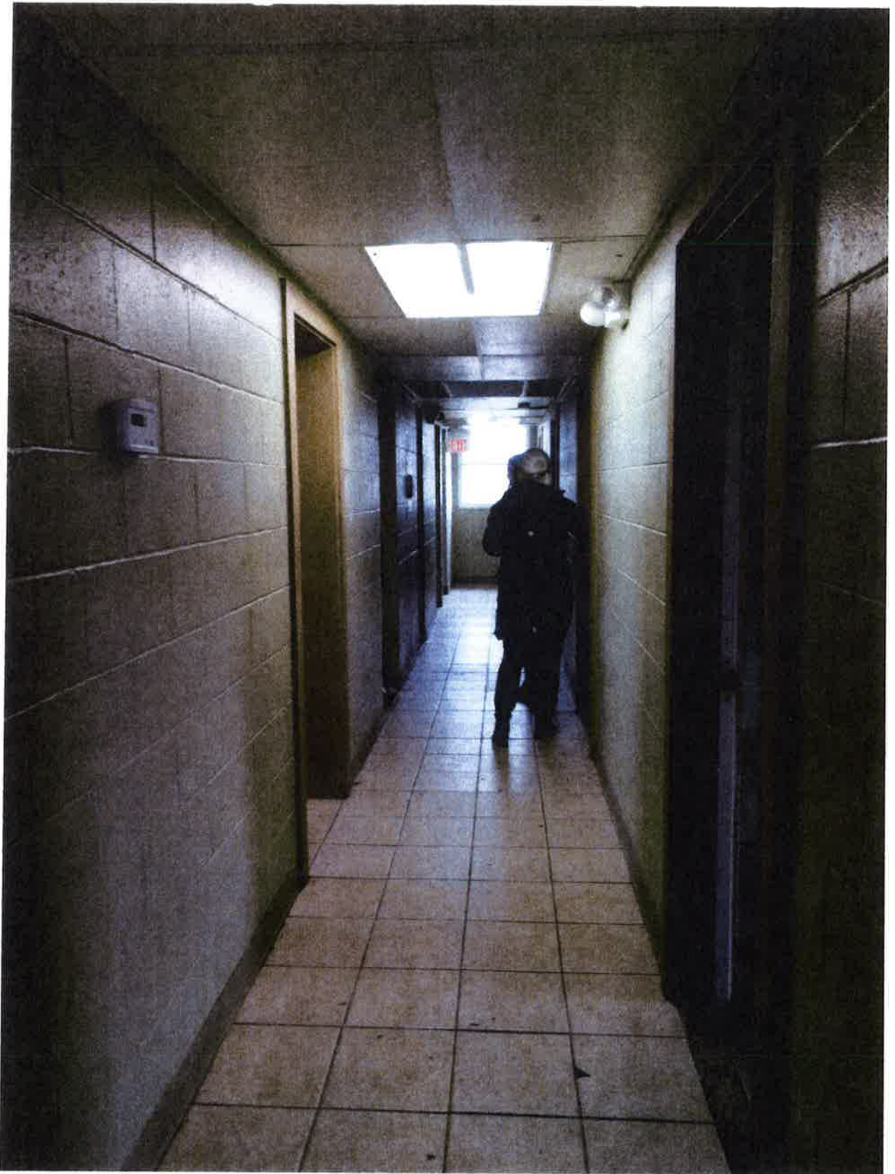
Second Floor Hallway
