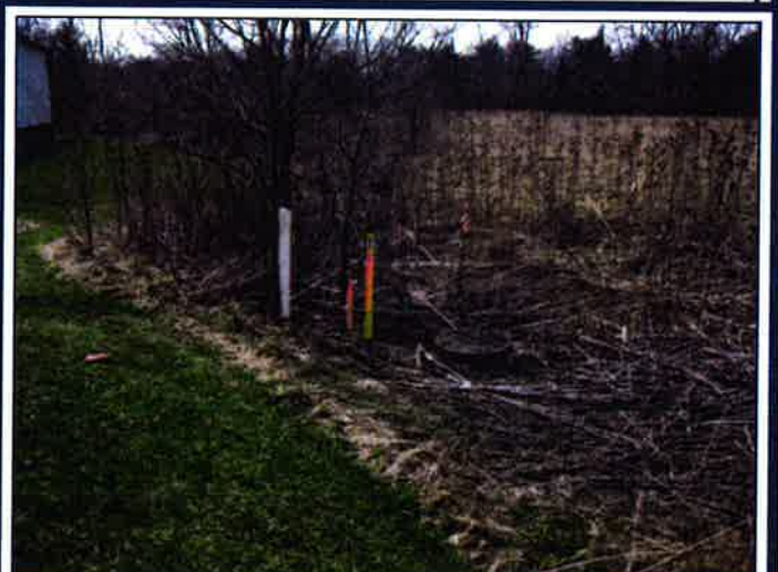
8 - Sanitary Sewer MH Near South Corner
