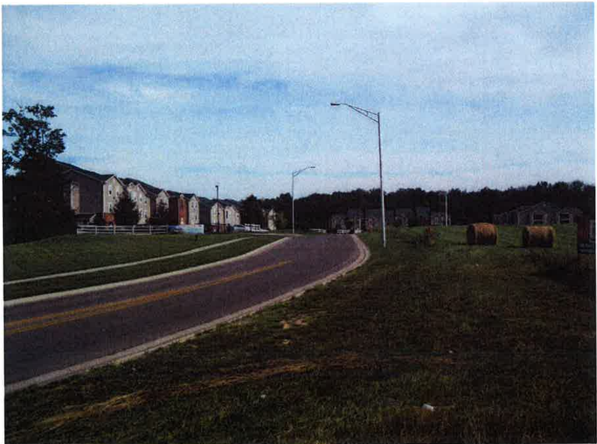
(4) View from proposed main entrance of Collegiate at Oxford looking north along Southpointe Pkwy. towards Level 27 Apartments.
