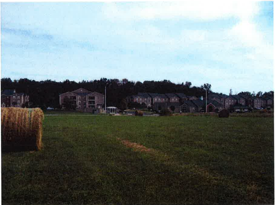
(8) View from the center of the subject site looking north.
