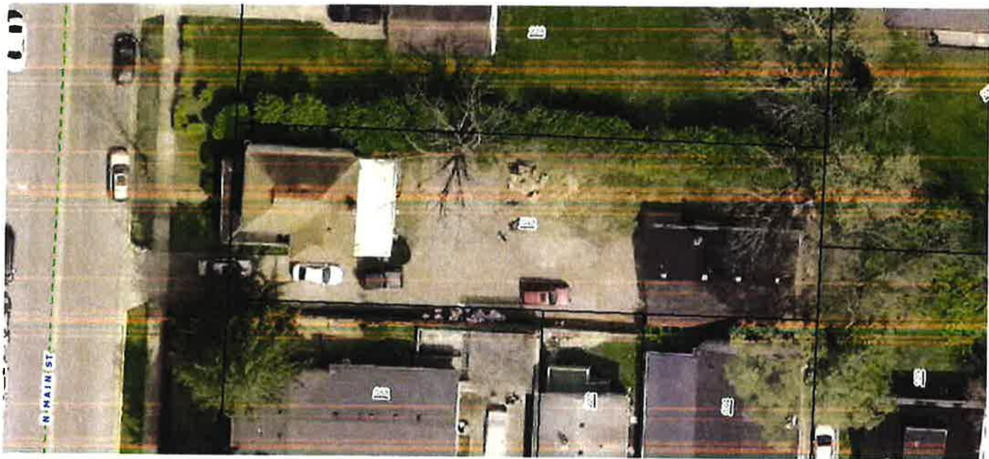
Aerial View showing relationship between main house and existing accessory building
