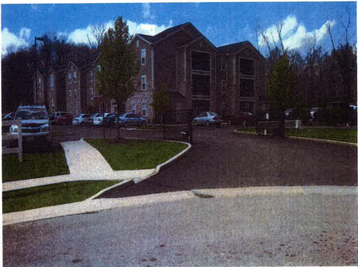
(24) View from the cul-de-sac of Corporate Woods Lane looking west into Level 27 apartments.
