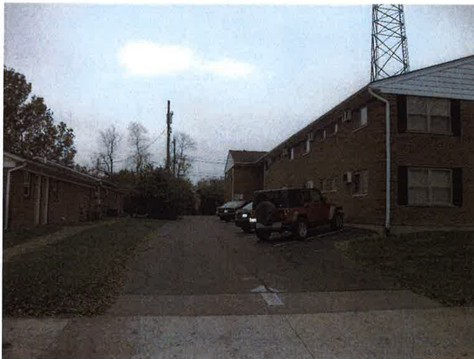
View from the center of Arrowhead Dr. at the south property line facing southwest along existing building #4
