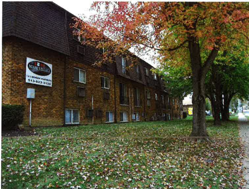
View from the corner of Chestnut St. and Arrowhead Dr. facing southwest towards existing building #1
